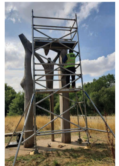
Peterborough Arch repair work
