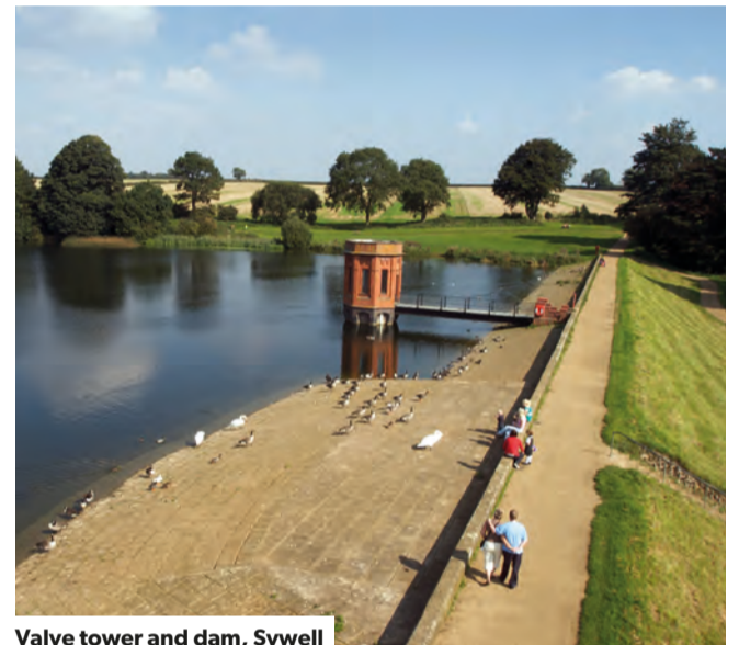
Valve tower and dam, Sywell
